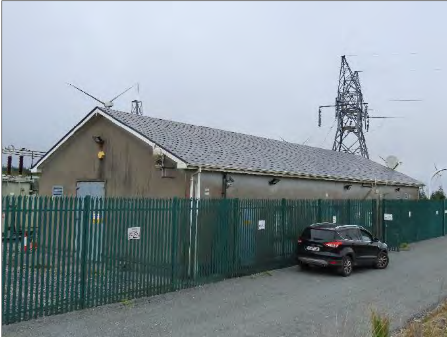
Photograph 2: Derrybrien Substation building (south elevation)
