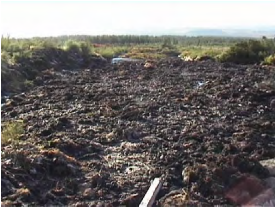
T17 - East of Turbine Base Looking Downslope of Failure.
