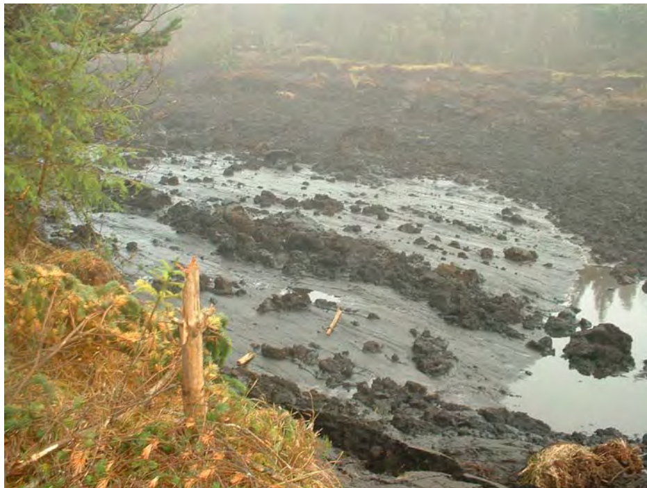
T68 – Failure Plane Approximately 50m South of Base.
